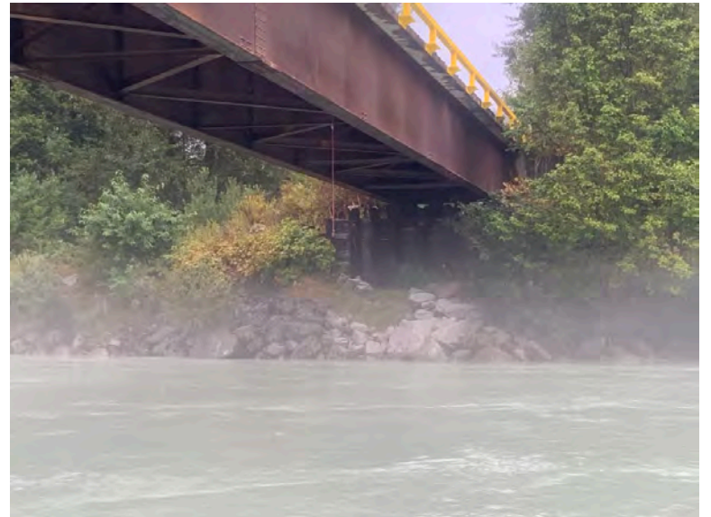
Left Bank Abutment when facing downstream
