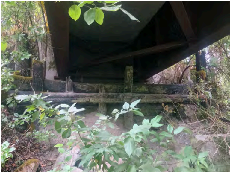
Right Bank Abutment when facing downstream
