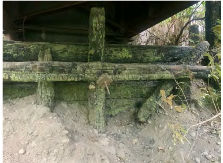
Right Bank Abutment when facing downstream
