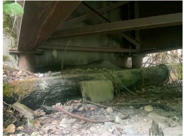
Right Bank Abutment when facing downstream
